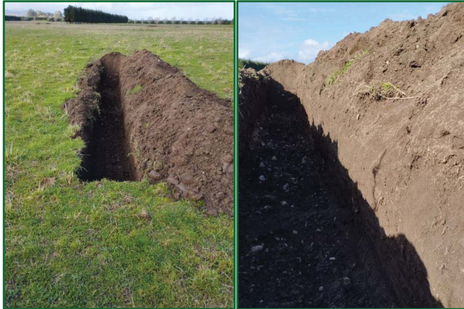
Photo 15 & 16 – Test pit location 24
