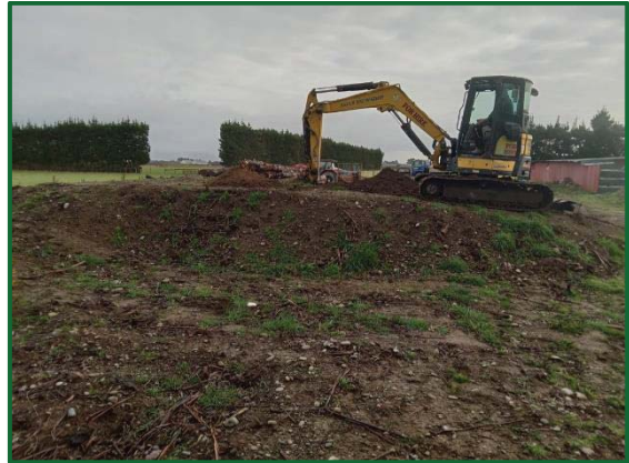
Photo 6 – Test pit location 7
