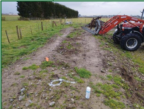
Photo 7 – Test pit location 9
