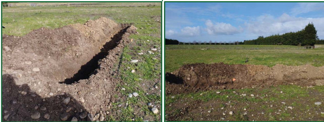
Photo 17 & 18 – Test pit location 25
